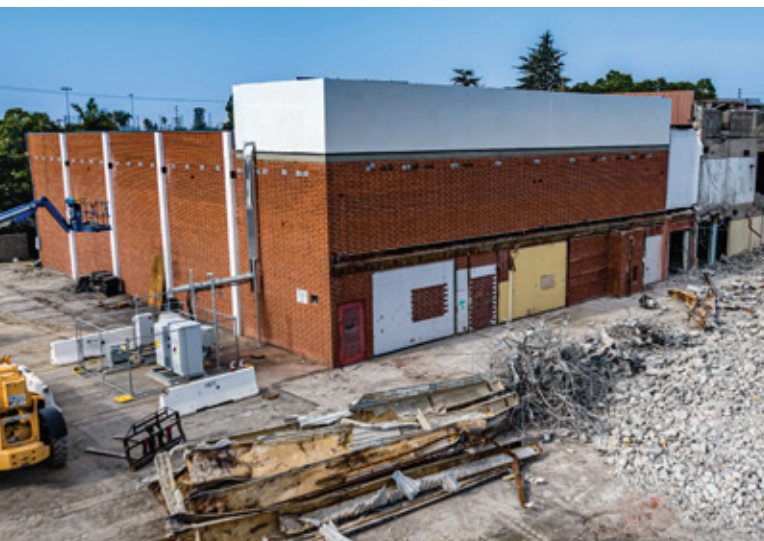
Construction in progress
